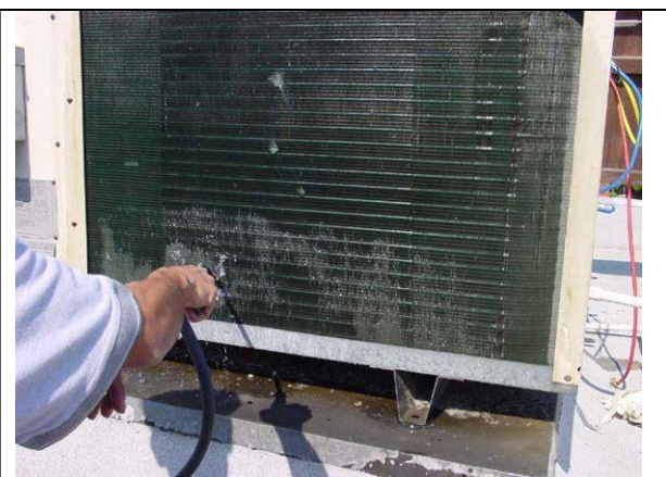
Figure 2.2 Cleaning Tube & Fin Condenser
