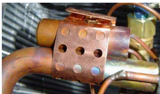
Figure 1.4 TXV Sensing Bulb with Copper Strap at Correct Position on Suction Line
